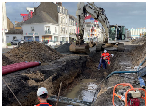
The repair work on the heavy-duty roadway will end in March.
