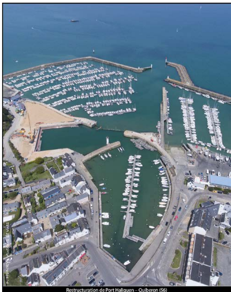
Restructuration de Port Halgouen – Quiberon (56)
