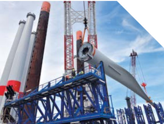
Wind turbine blades being loaded.
