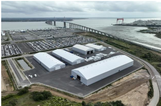
In the space of two years, five metal-and-textile buildings have been delivered at the industrial operations facility.
