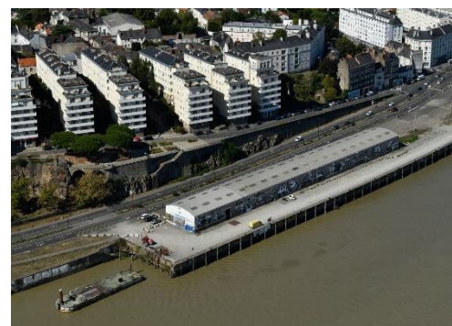
The site of Shed 12, Quai d'Aiguillon, is forming the subject of a real-estate development project.
