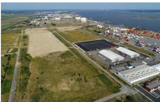
Areas that are subject to the constraints of the TRPP are being utilized for the installation of photovoltaic power plants at Montoir de Bretagne.
