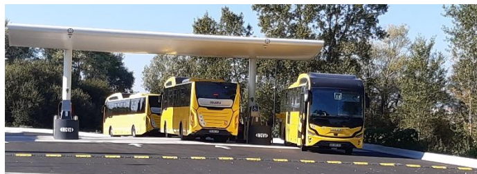
The NGV station GNV at Montoir de Bretagne.
